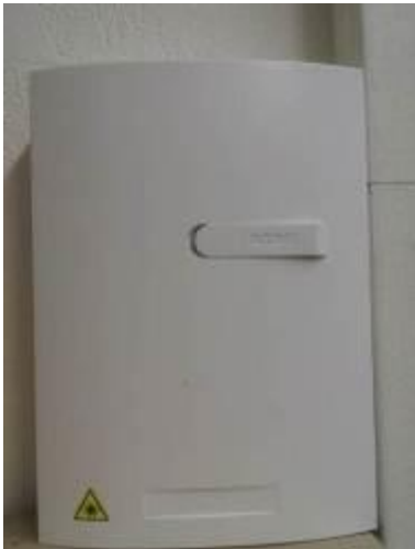
Figure 10 : PBO ACOME mono fibre
